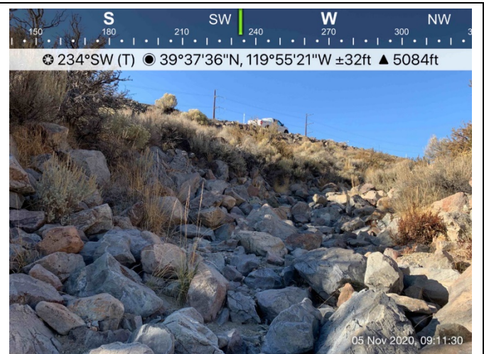
Photo 2. Riprap lined intermittent stream (D-7c). Intermittent streams were documented in D-1 with data point 1.
